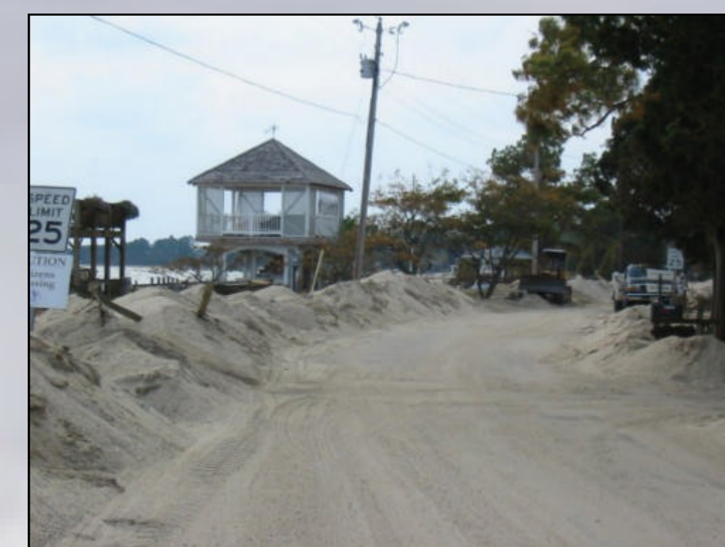
Bulldozers removed several feet of sand transported from the beach to a nearby road. Piney Pt., Potomac R., St. Mary's Co. [10]
