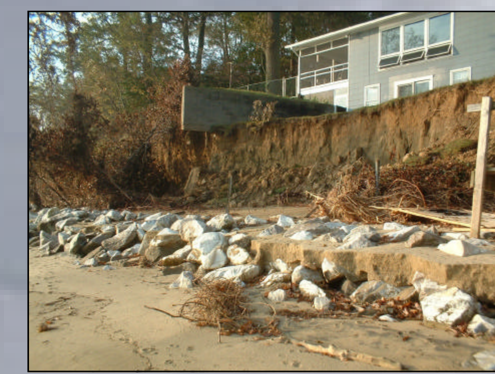
Based in part on images like this, MGS assumed that, along eroded shorelines, a 5-ft high bank retreated 5 ft. Annapolis Roads, Chesapeake Bay, Anne Arundel Co. [2]
