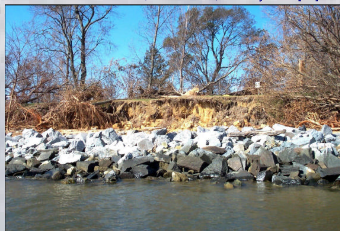
Bank erosion due to vertical expansion of zone of wave influence. St. Clements I., Potomac R., St. Mary's Co. [10]
