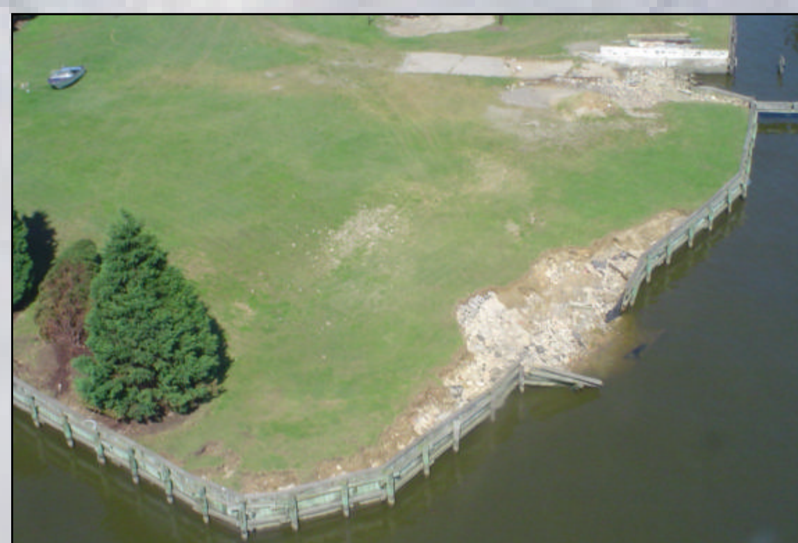
Bulkhead failure and fastland scour associated with storm surge ebb. Chesapeake Bay, Baltimore Co. [11]
