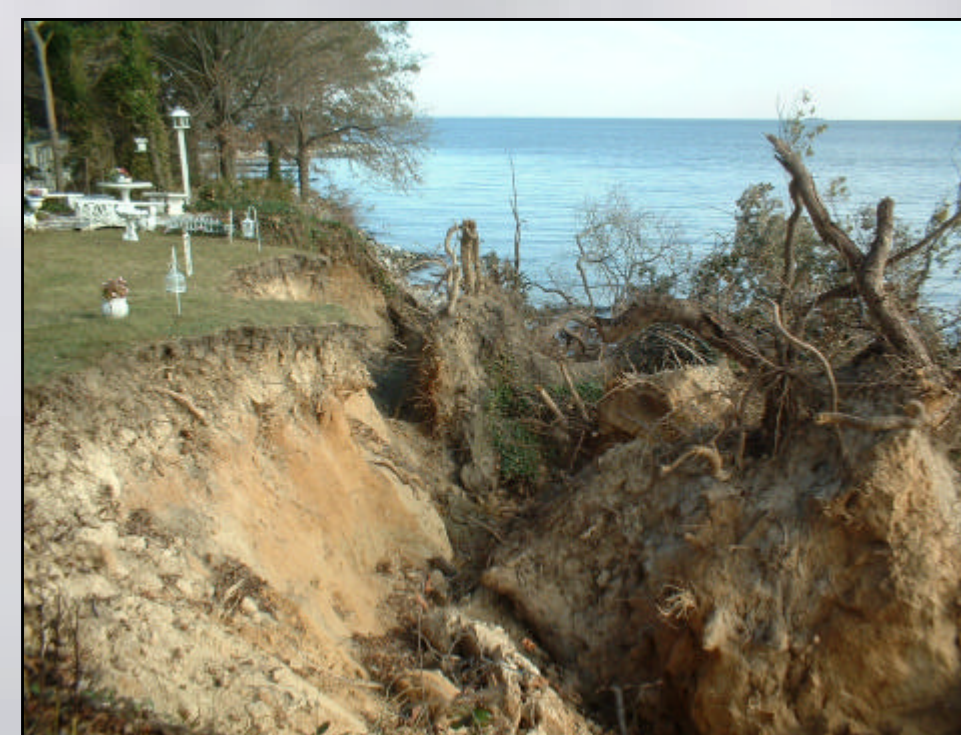
Slope undercut by floodwaters overtopping 2-3 ft stone wall and undermining mature trees. Gibson I., Chesapeake Bay, Anne Arundel Co. [2]
