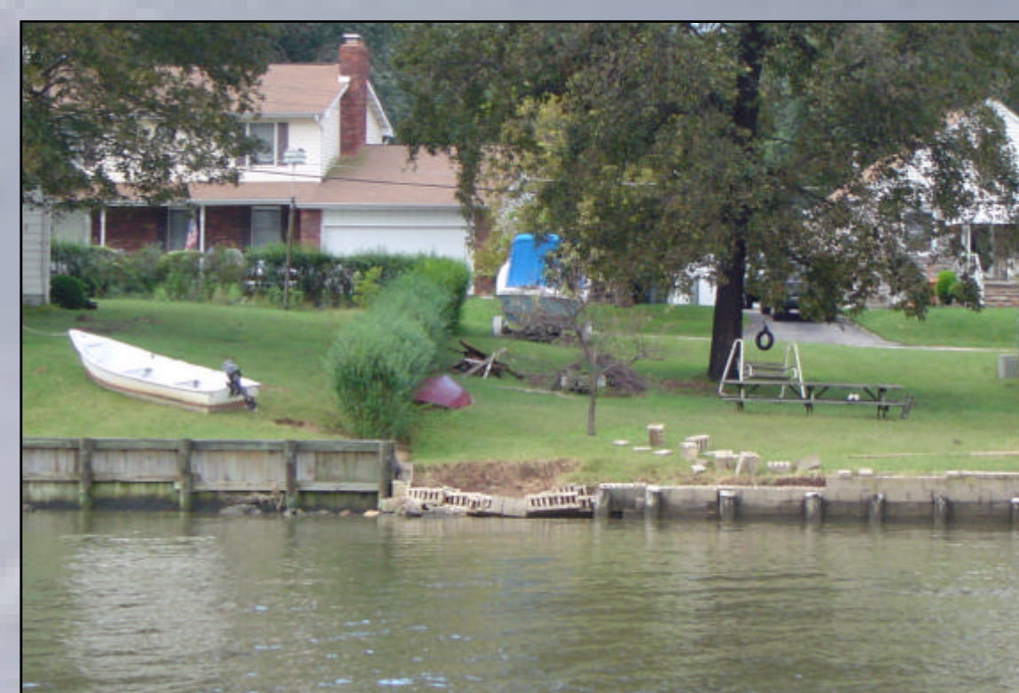
Effects of storm surge flood (cinder blocks carried inland) and ebb (collapse of block wall; scour near motor boat). Middle R., Baltimore Co. [11]
