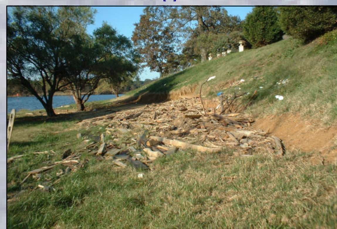
Erosion of inland bank due to lateral expansion of zone of wave influence. Anne Arundel Co. [2]
