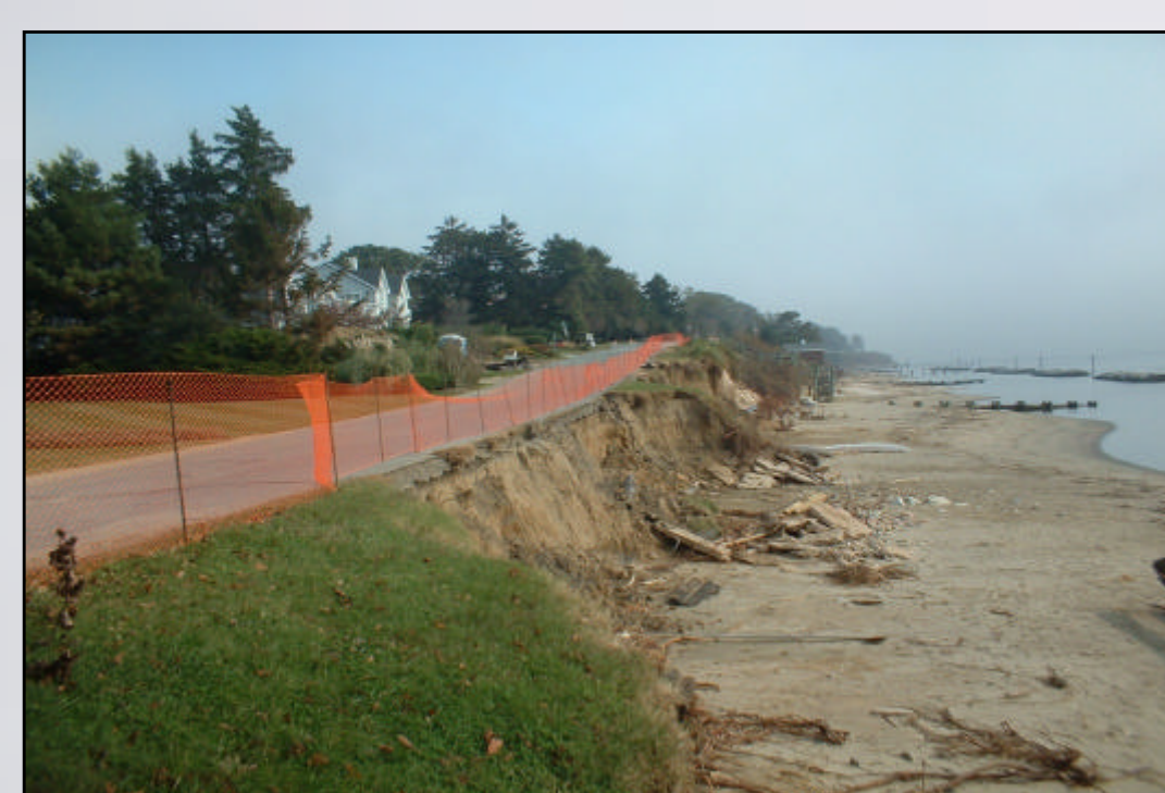
Severe erosion threatens road. Bay Ridge, Chesapeake Bay, Anne Arundel Co. [2]
